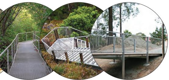
A steel elevated walkway down the slope would allow minimal disruption to roots and storm water flow down the hillside while providing great opportunities for views. In this application most sections would not require a full balustrade, just a handrail.
