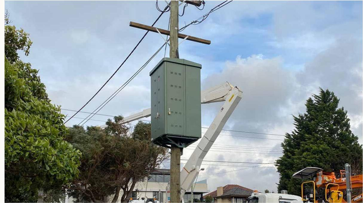
*Figure 3. Image from RenewEconomy, 2021, Hanging batts: 40 pole-mounted community batteries to boost grid reliability*
